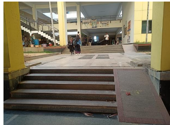
Ramp at the bifurcation between NA-Block, and NB-Block
