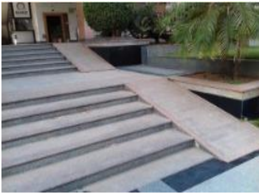
Ramp at NA-Block Entrance
